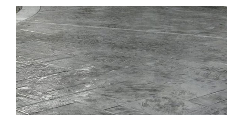
PATIOS - GULL GRAY CONCRETE WITH DEEP CHARCOAL RELEASE/ SLATE GRAY SHAKER HARDENER
